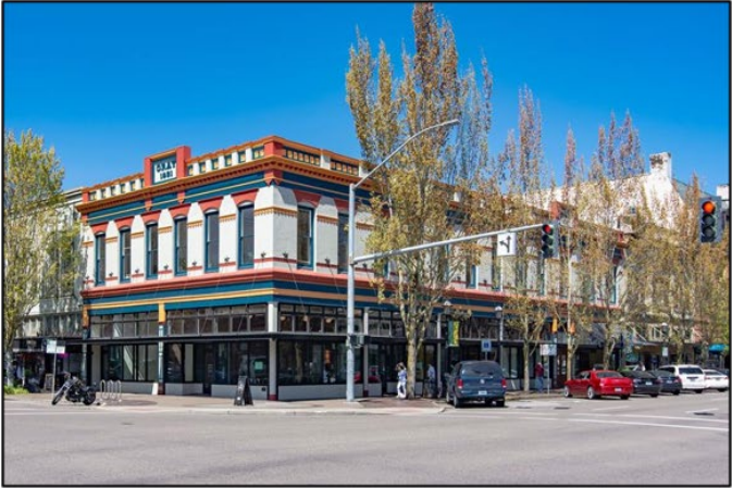
Gray Building (105-135 Liberty Street NE, Salem, OR) Lowest image shows the rehabilitation of historic awning configuration from circa 1912. (Sources top to bottom: Willamette Heritage Center, Google Streetview 2012, City of Salem)
