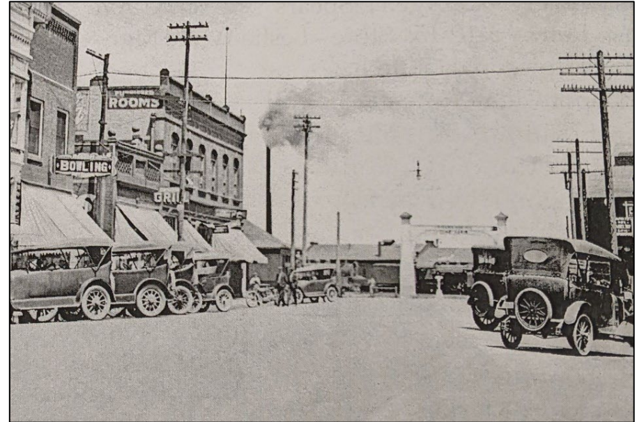
View of Depot Street with a freestanding arch in the background leading to the railway station, c.1926-28 (Source: RPB Collection)
