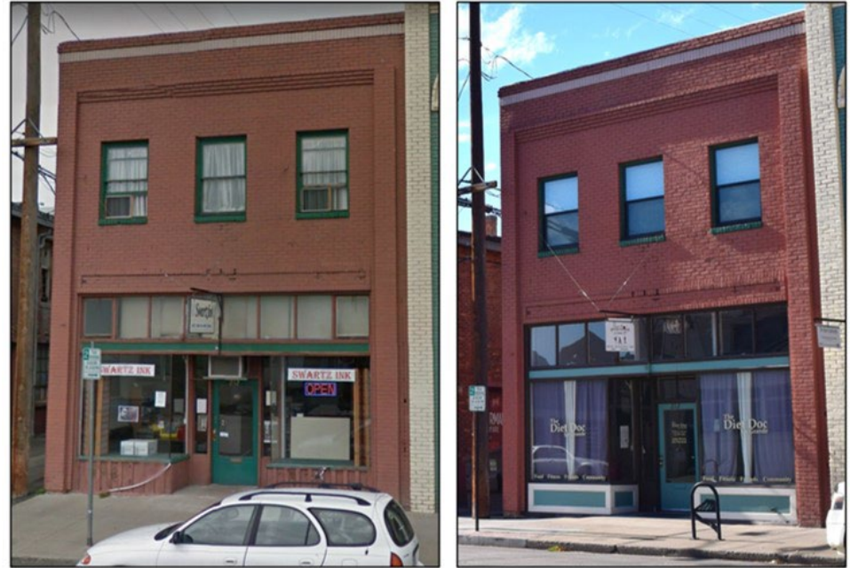
212 Fir Street is a good example of a rehabilitated storefront. Note the new panelized bulkhead beneath the storefront windows. (Source for image on left: Google Street View 2012)
