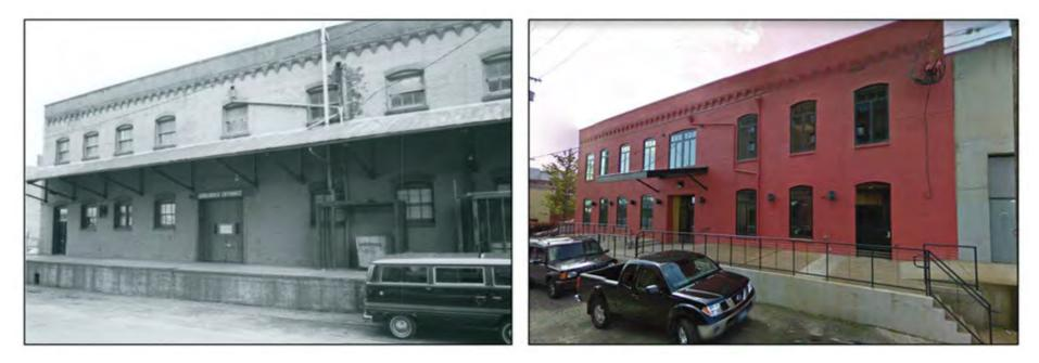
This former warehouse building was rehabilitated for a new use circa 2008. Alterations included the replacement of the small loading dock windows with larger windows. A full storefront bay expression would have conveyed the wrong "story" about the building's original use. This style of rehabilitation could be applied to buildings along Jefferson Avenue. (Source for image on left: c.1980 City of Portland Historic Resource Inventory) (Source for image on right: 2009 Google Street View)
